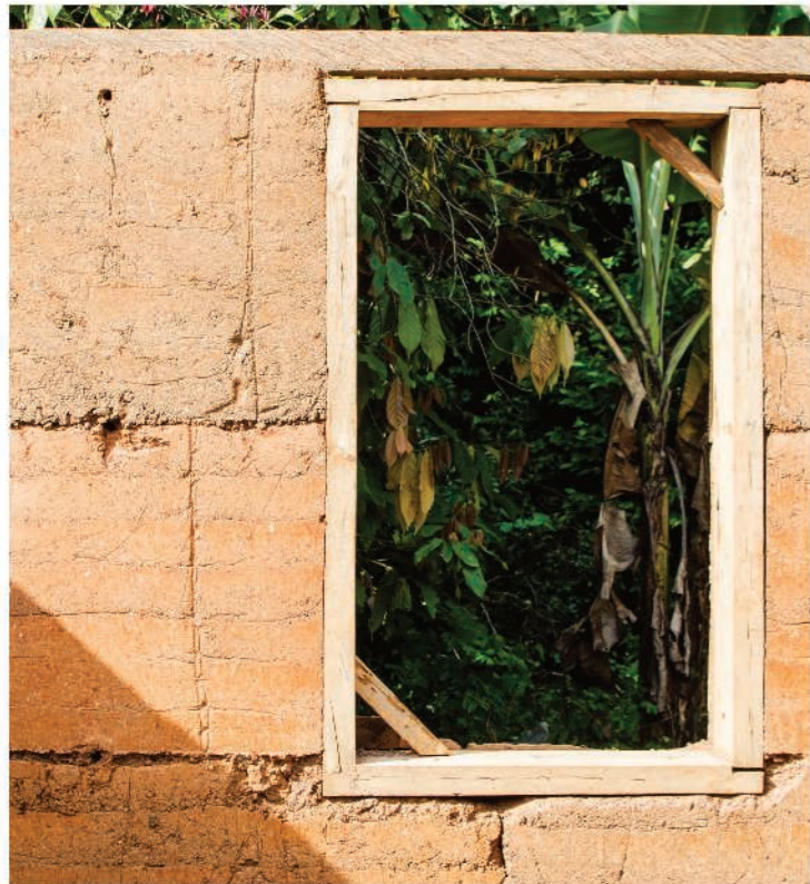
1. Opoku's house walls front view
