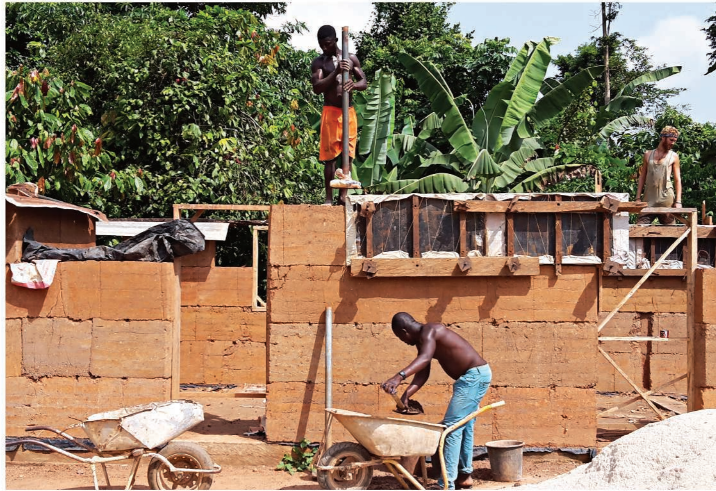
1. Detail of the rammed earth wall of the back side
