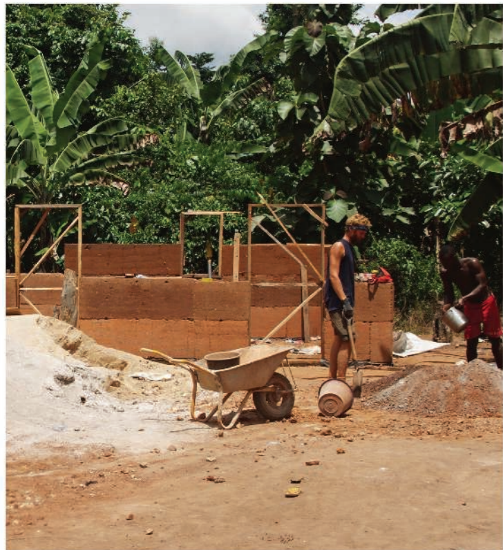
1. Detail of the rammed earth wall of the back side
